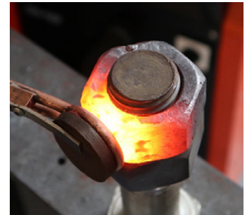
› Preheating before welding
